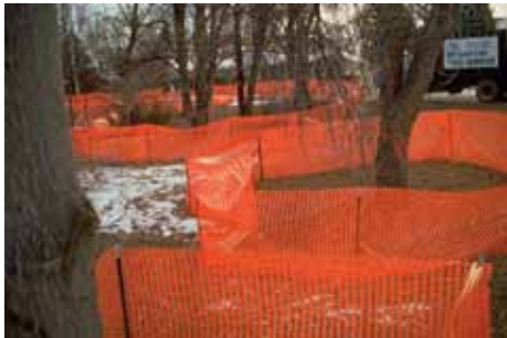
Figure 2: Highly visible tree protection barriers.
