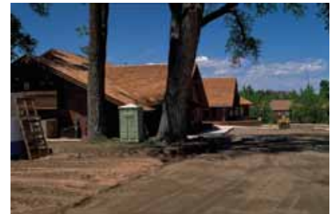
Figure 4: Surface grading severs many roots.
