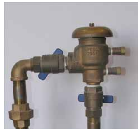
Figure 4: Both ball valves and test cocks should be exercised back and forth several times.
