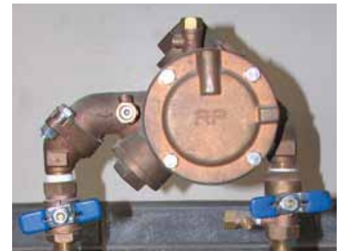
Figure 4: Reduced Pressure Device.
