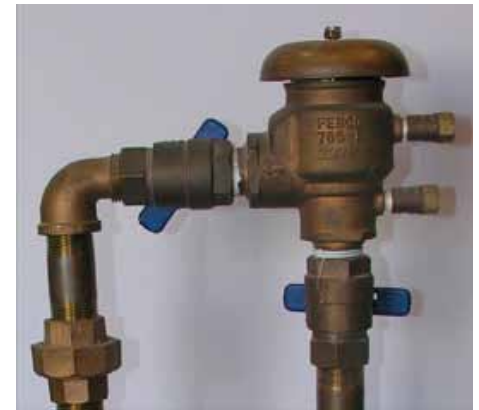
Figure 3: Pressure Vacuum Breaker.
