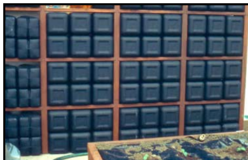
Figure 2. Milk jug water storage wall in a passive solar hobby greenhouse – Disposable milk jugs on left and returnable milk jugs on right are spray painted flat black. In this well-built structure, nighttime temperatures dropped to 39° with no supplemental heat when outside temperatures dropped to minus 17° F.
