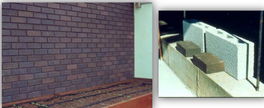
Figure 1. Brick storage wall in passive solar hobby greenhouse – Thermal storage mass is a wall made with two layers of brick filled with concrete. In this well-built structure, nighttime temperatures dropped to 35°F with no supplemental heat when outside temperatures dropped to -17°F. Note young crops in raised-bed style garden with drip irrigation.
