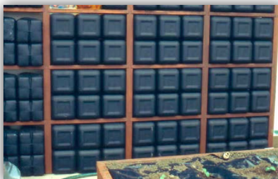
Figure 2. Milk jug water storage wall in a passive solar hobby greenhouse. Disposable milk jugs on left and returnable milk jugs on right are spray painted flat black. In this well-built structure, nighttime temperatures dropped to 39°F with no supplemental heat when outside temperatures dropped to -17°F.
