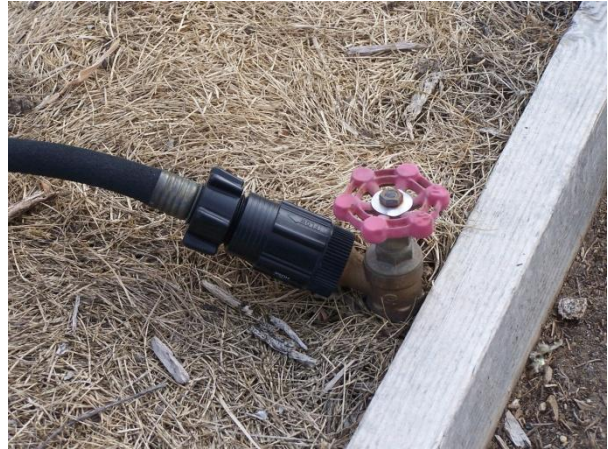
Figure 4. With irrigation pipe, it is easy to plumb a tap at each raised bed box. Here a pressure regulator with hose-end fittings reduces pressure to 25 psi. It is connected to a ½-inch soaker hose.
