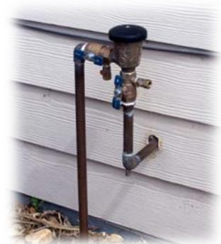
Figure 2. Required by local building codes, backflow prevention devices are typically located where the line comes outside from the house.
