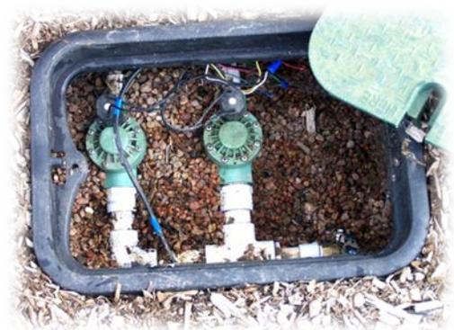
Figure 3. Valve box with two zone valves.
