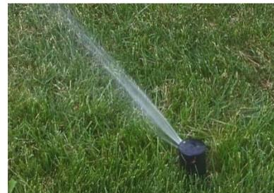
The spray pattern depends on the head. Most can be set at any angle from 15° up to a full circle. Some are adjusted at 15° increments. Others are designed for a quarter-circle, half-circle or full-circle spray pattern.
