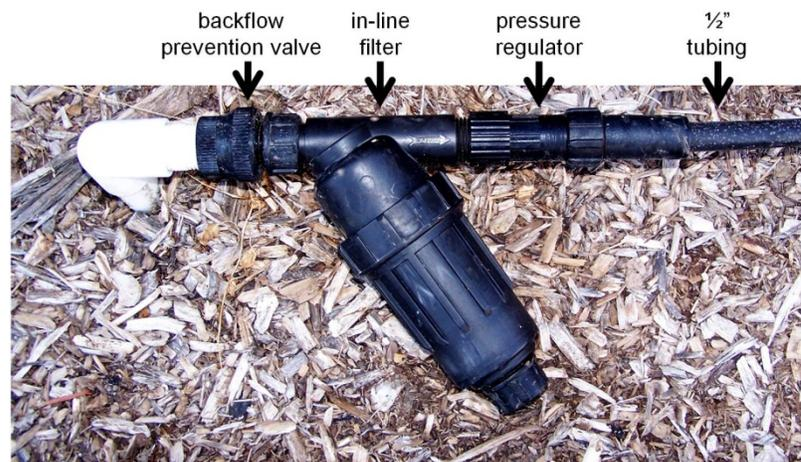
Figure 9. In-line filter and pressure regulator going to drip line poly tubing.
